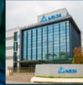
Chungli R&D Building LEED Gold
