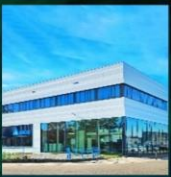
Helmond Office LEED Gold
