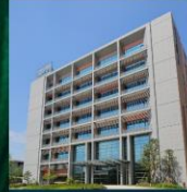
Taoyuan Plant 5 LEED Gold EEWH Gold
